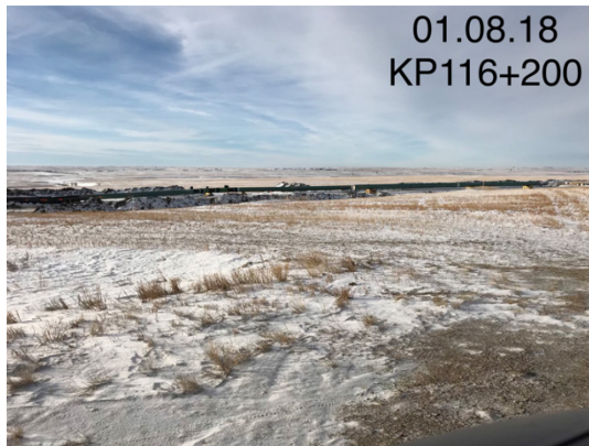
1. Pipe on skids - Km 116+200 – Jan 8, 2018
