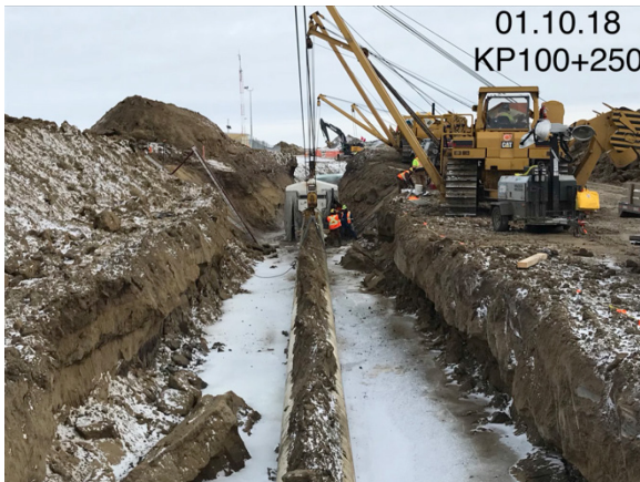
9. Re-excavated tie-in – Km 100+250 – Jan 10, 2018
