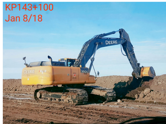
2. Backfill – Km 143+100 – Jan 8, 2018
