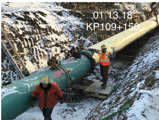
21. Booms picking up pipe - km 109+150 – Jan 13, 2018
