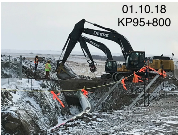
9. Re-excavated tie-in – Km 100+250 – Jan 10, 2018
