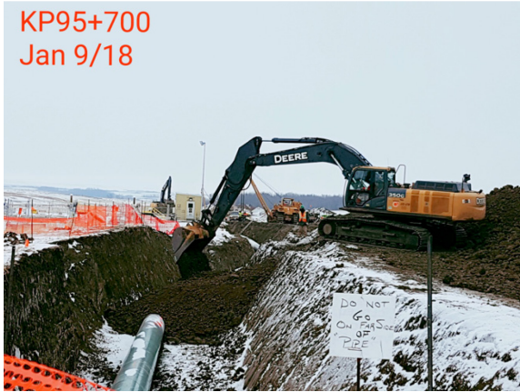
7. Track hoe backfill – Km 95+700 – Jan 9, 2018
