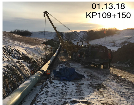
22. Side booms moving pipe – km 108+950 – Jan 13, 2018
