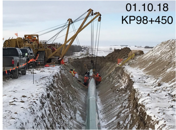
8. Tie-in backfill – km 98+450 – Jan 10, 2018
