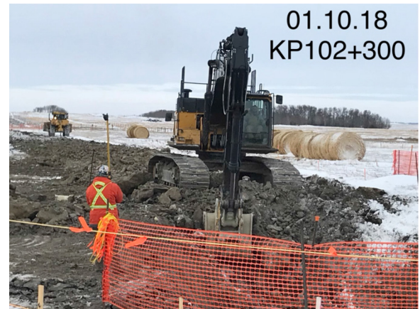
10. Digging in bell hole – Km 102+300 – Jan 10, 2018
